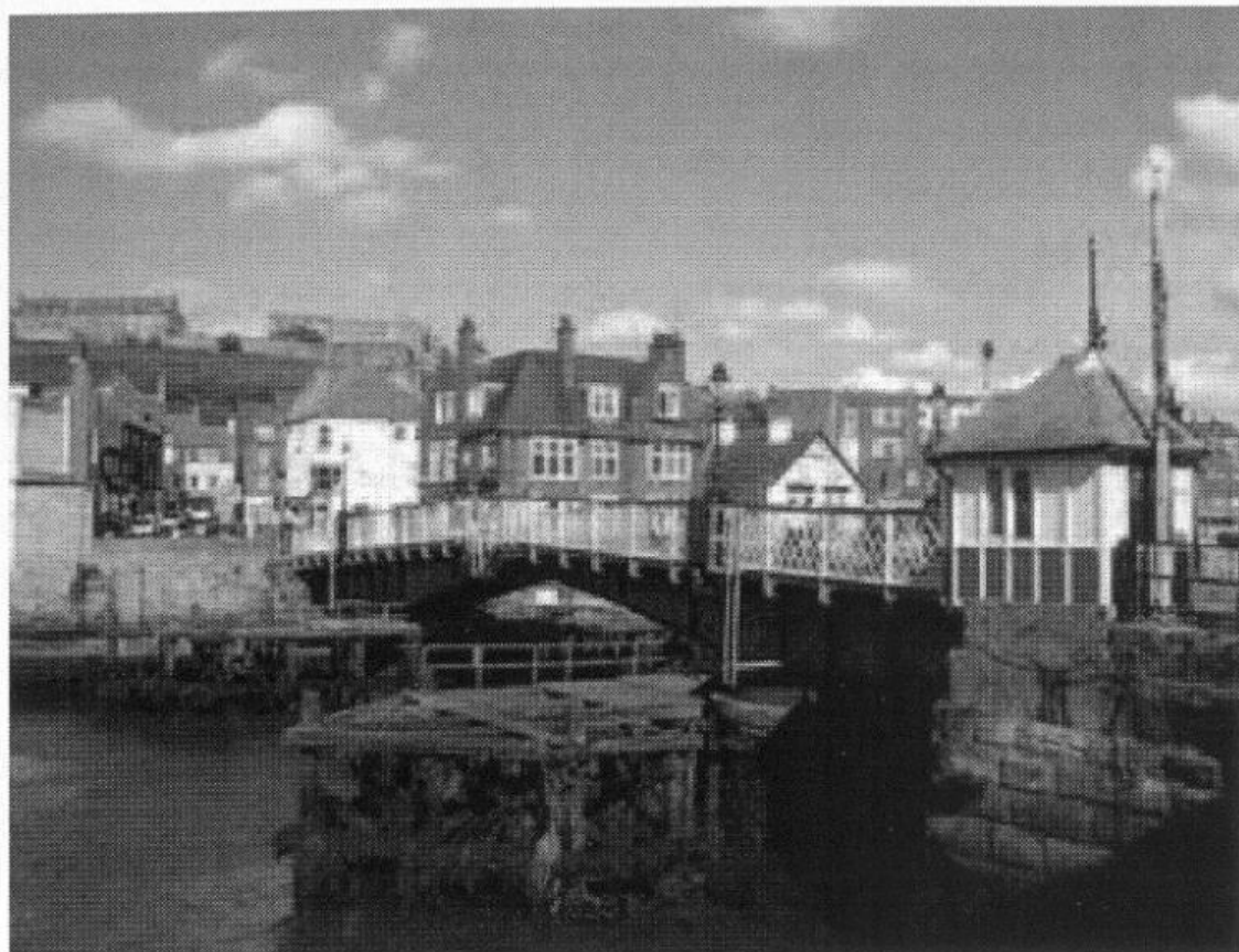
1908 swing bridge across the river Esk, near the harbour,
